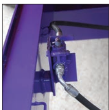
Hyd Door Safety Valve
